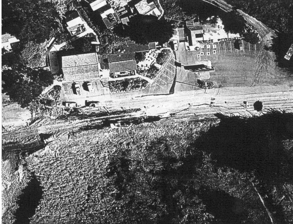
Aerial view of landslide at Gorda, January 2, 1997 (Photograph reprinted from: Caltrans Annual Report, 1997/1998 )
